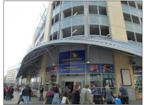
Entrance to the Bullring Indoor Market
