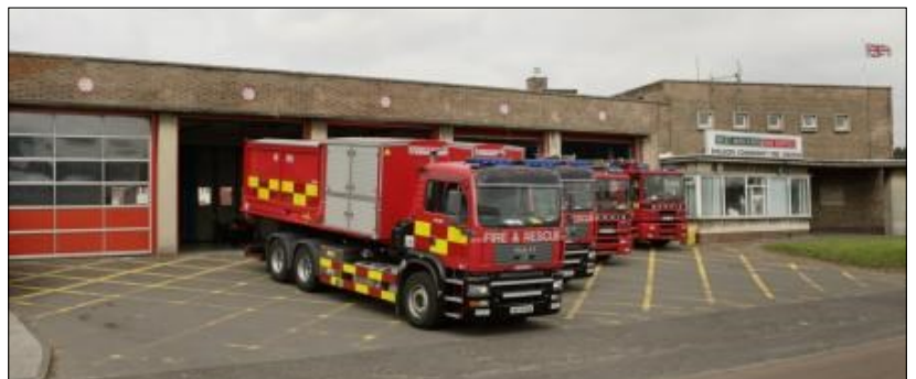
Sheldon Fire Station
